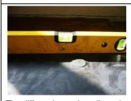
The diffuser has to be adjusted horizontally before the clamp is finally tightened.
